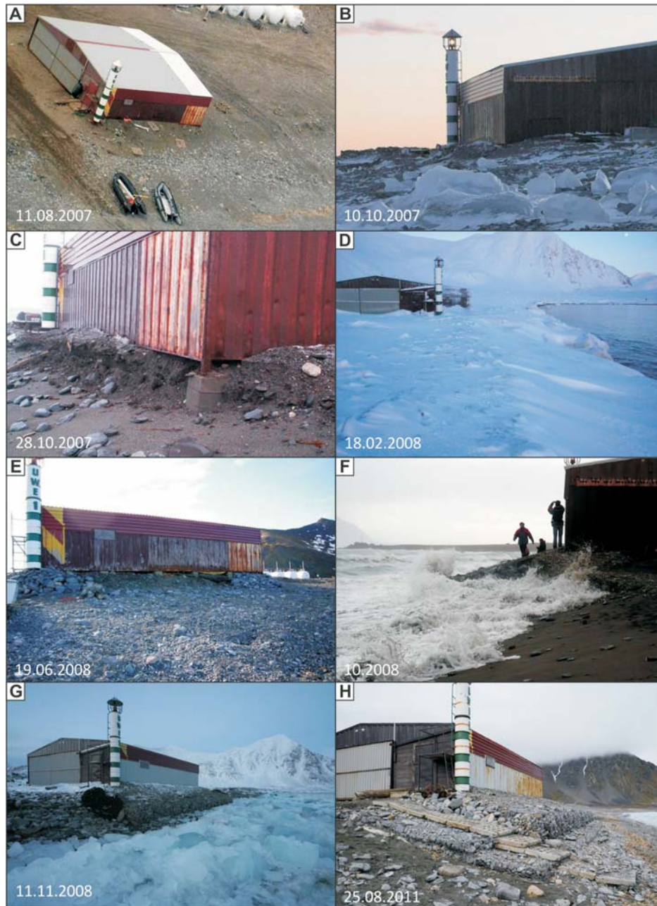
Fig. 8. The effects of coastal erosion processes in the area of harbour building of Polish Polar Station – “Banachówka” and methods of its protection. Photo: M. Błaszczuk archive (A–D, F), J. Kwaczyński (E, G), P. Zagórski (H).
