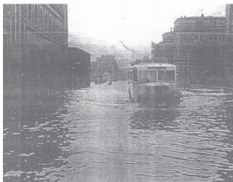
Figure 8. Gliwice during the 1940 flood – Krakowska Street area.
