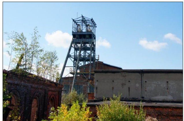
Fig. 2. "Klara" shaft in abandoned mine "Wawel" (K. Mazurek)
