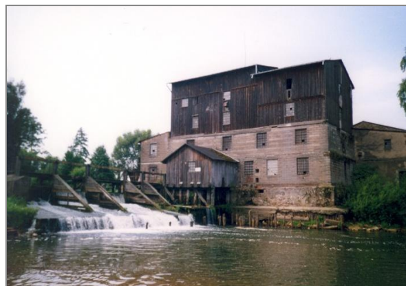
Fig. 3. Marcelin mill in Krzepice (before weir renovation) (M. Fajer)
