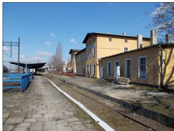
Fig. 3. The railway station building in Mysłowice, 2014 (W. Dragan)
