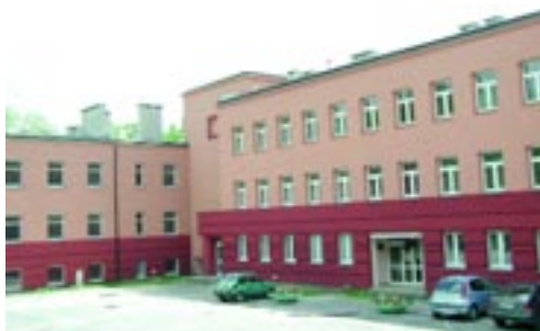
Fig. 1. New building of the Scientific Herbarium of the University of Silesia (KTU).
