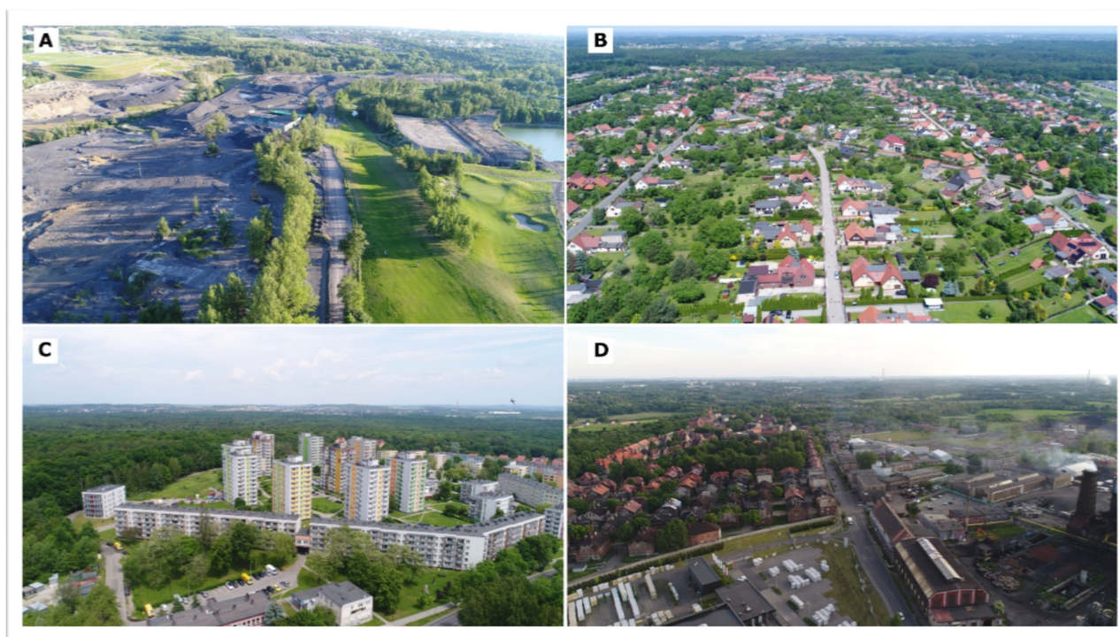
Figure 7. Selected landscapes of Bytom in 2021 (Sourced by authors). Explanations: (A)—Reclaimed areas of the former the Szombierki Coal Mine; (B)—Single-family housing in the agricultural district of the Stolarzowice; (C)—Housing estate in the Miechowice district; (D)—The workers' housing estate from the beginning of the 20th century (Nowa Kolonia Robotnicza) and a coking plant in the Bobrek district.
