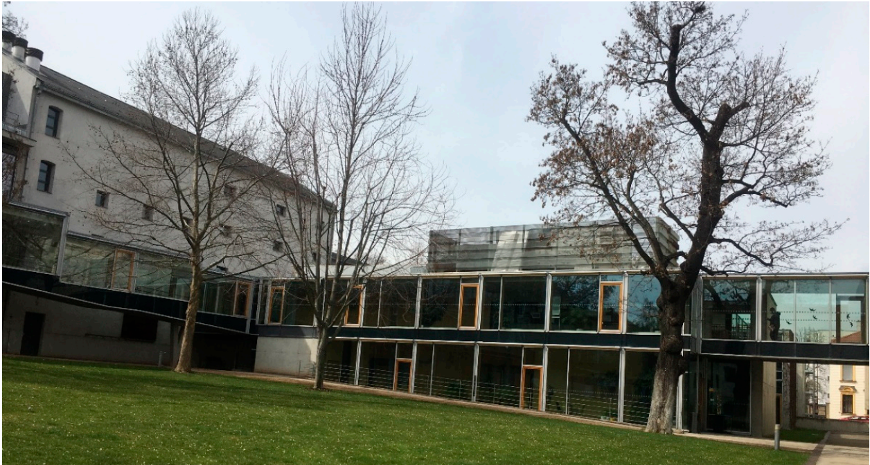
Figure 7. Rebuilt former malt house incorporated into new modern architecture to meet the needs of the Faculty of Information Technology, University of Technology (Photo: K. Charvátová).
